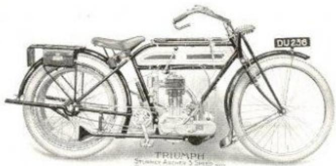
STURMEY-ARCHER THREE-SPEED GEAR MODEL WITH TRIUMPH GEAR AND CLUTCH CONTROL.
